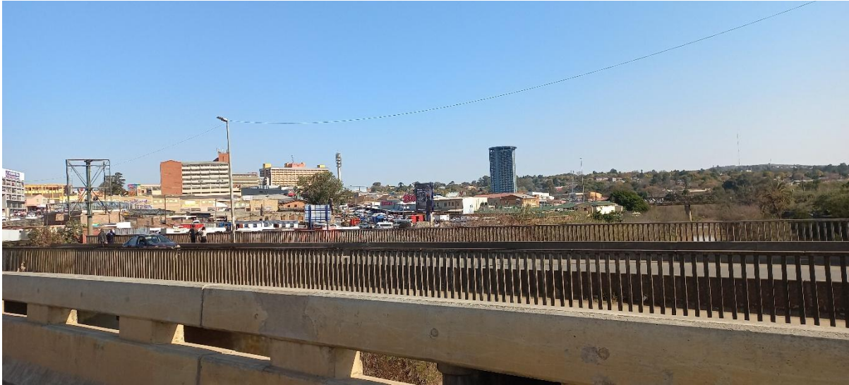
Figure 8-17: Bridge Leading into uMthatha Town
