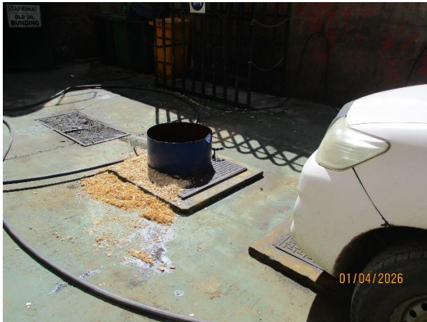
Photo 1: Wash bay with drain to oil sump.
