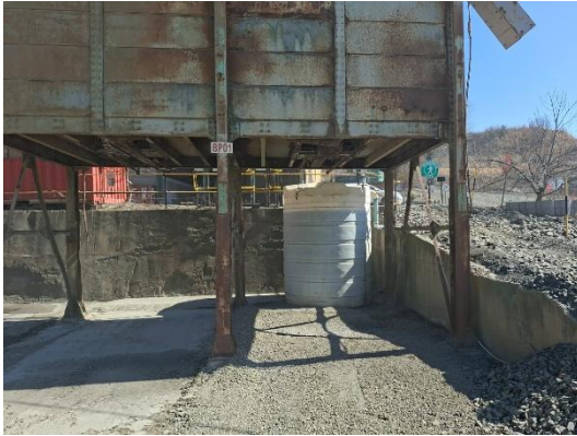
Photo 7: JoJo Tank storing "clean water" from the oil sump located in the wash bay.
