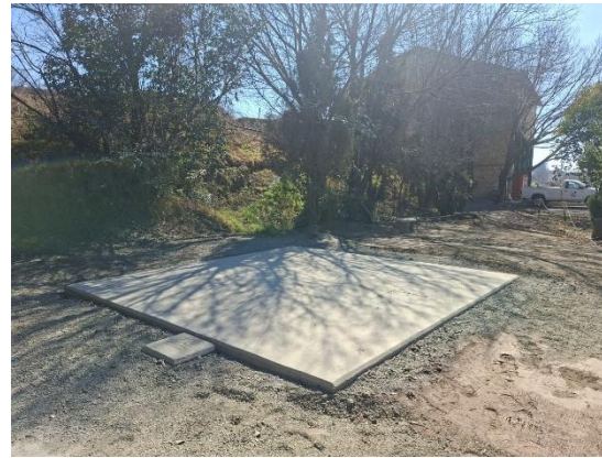
Photo 8: Conservancy tank attached to the change house ablution facility.
