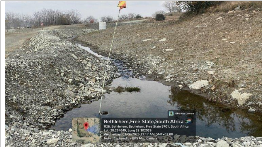
Photo C5: Existing ponding/retention condition requiring formalisation.
