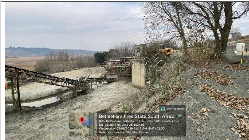
Photo C7: Ponding at worksite to be channelled to collection point.
