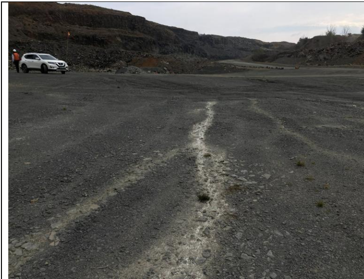
Photo C9: Dirty runoff pathway to retention pond.
