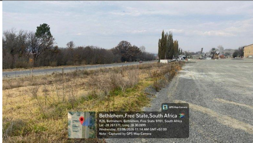
Photo C1: Roadside of storage area requiring berms.
