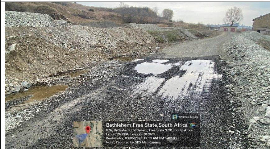
Photo C8: Ponding on roadways requiring regrading and drainage.
